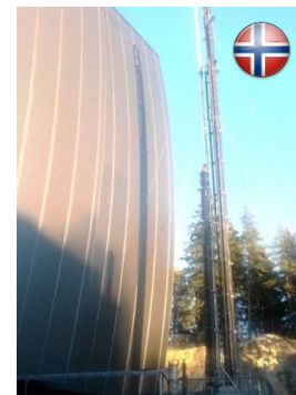
Waste to Energy Klemetsrud WtE
