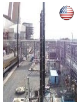
Coal National CCC
